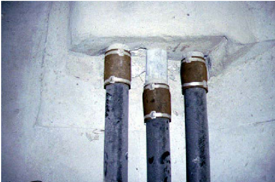
Figure 1.6: Plan View of Slipped Tendon at Deviation Saddle Niles Channel Bridge (FLDOT 2002)
