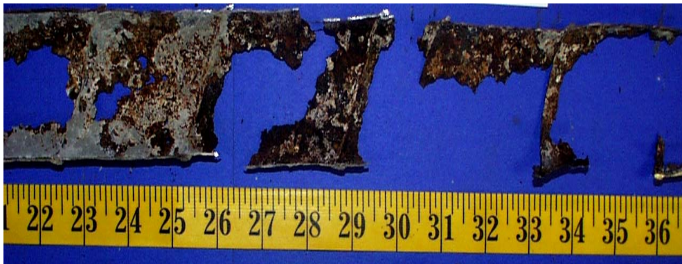
Figure 2.1: Corroded Galvanized Steel Duct (Breen and Kreger 2003)
