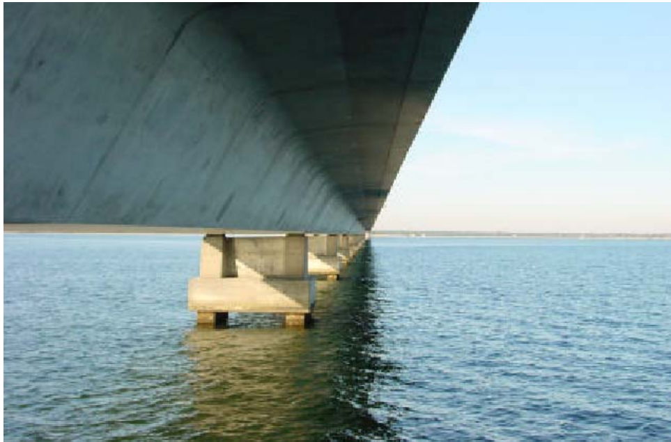
Figure 1.8: The Mid-Bay Bridge, Florida (FLDOT 2002)
