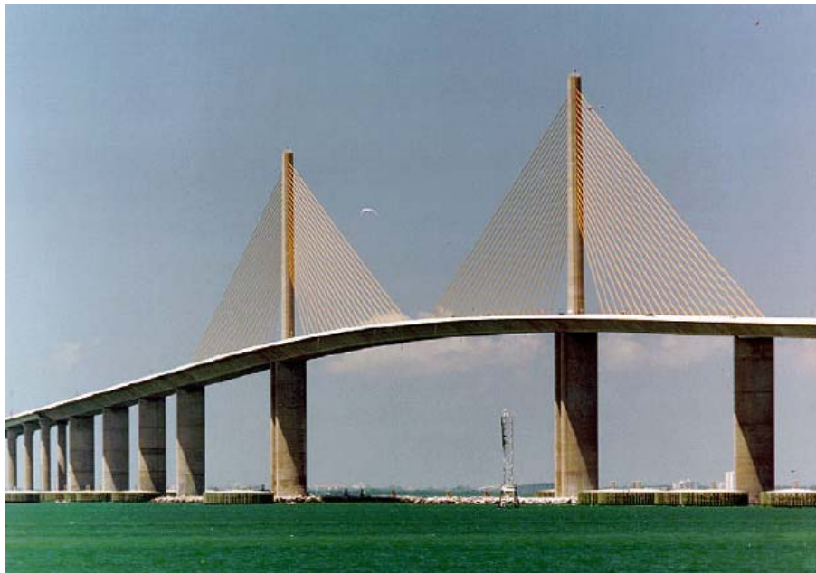
Figure 1.11: The Sunshine Skyway Bridge, Tampa, Florida (FLDOT 2002)
