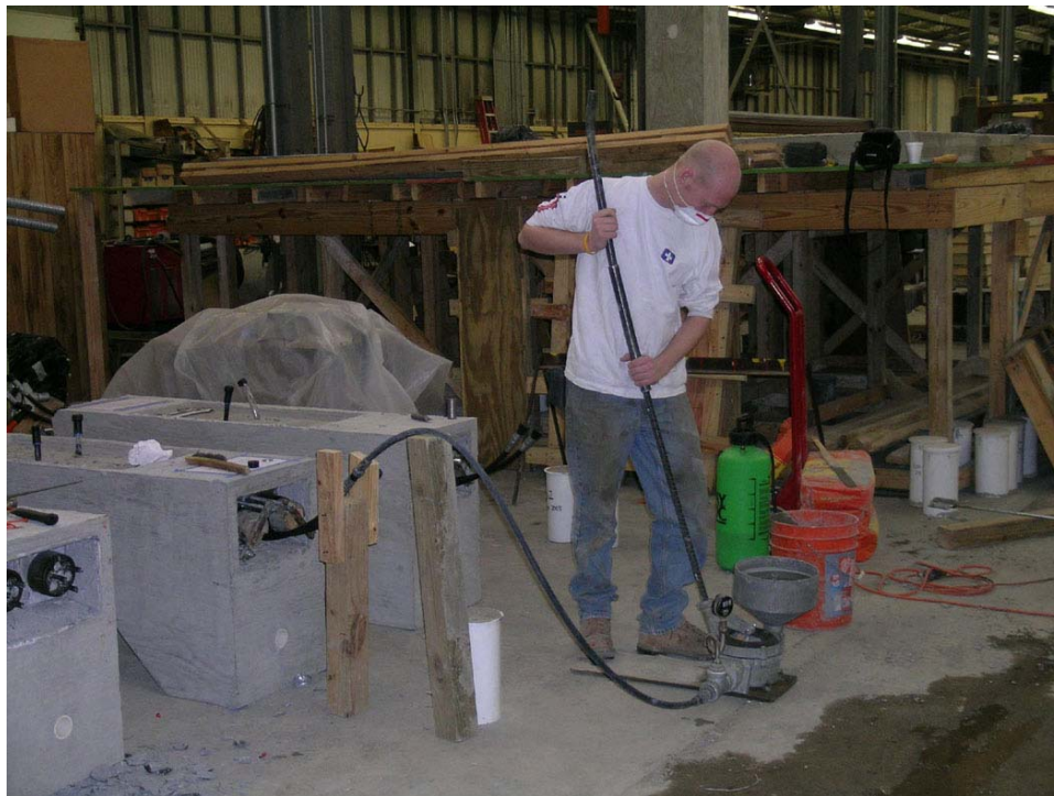
Figure 4.13: Grouting Specimens (Kyle Steuck pictured)
