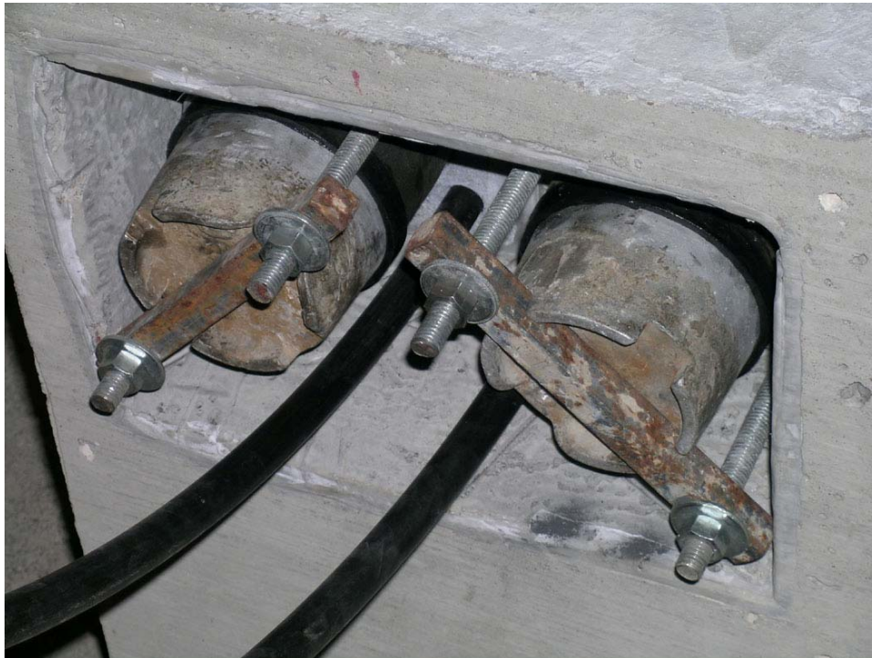
Figure 4.14: Temporary Grouting Caps
